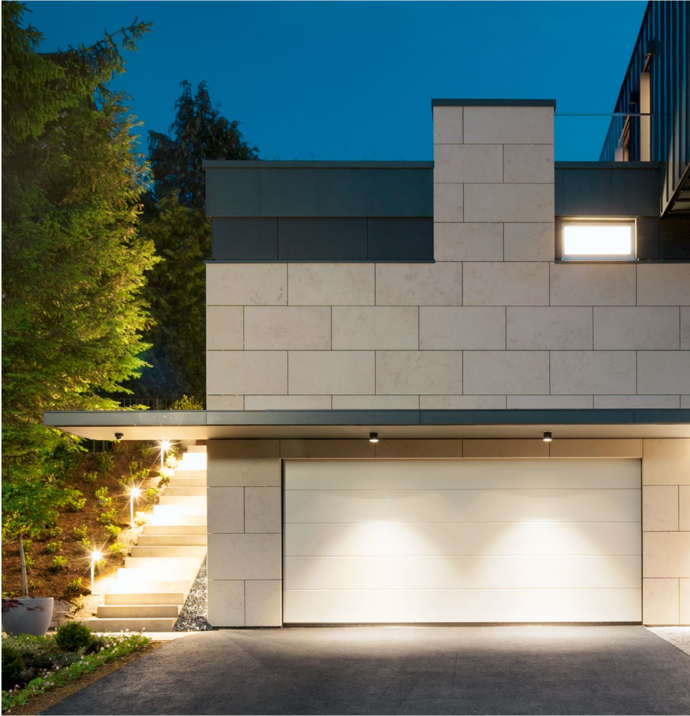
PRIVATE RESIDENCE | SPADO ARCHITECTS AUSTRIA
